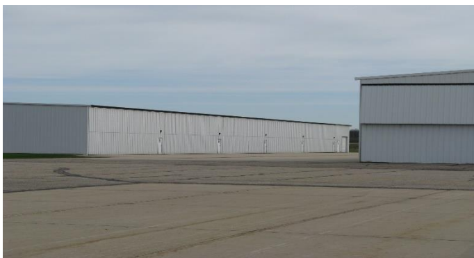
Photo: Existing T-Hangars (2021)
